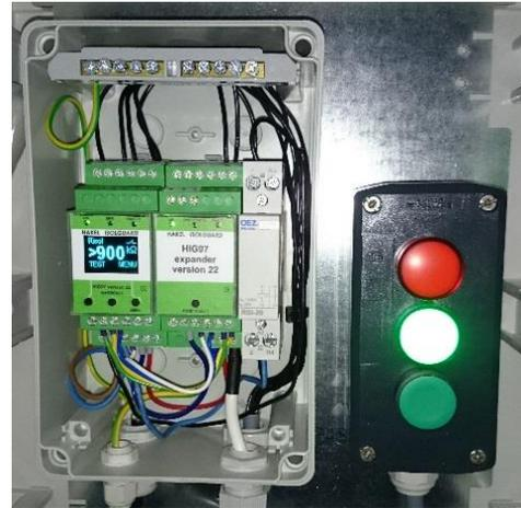
The HIG 97 IMD can communicate with a master computer via an RS485 industrial bus-bar by using a PROFIBUS-based protocol. The resistance range displayed is from 5 kΩ to 900 kΩ. Furthermore, the IMD includes 4 signalling relays. The ERR signalling relay signals the function of the IMD. As long as the insulation resistance device is OK and the insulation
