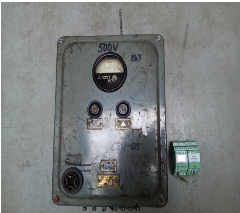
Fig. 3: Comparison between the previous CZU-05 IMD and the new HIG97 device
